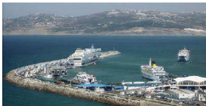
Port of Tanger Breakwater from W
