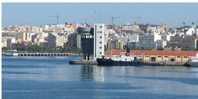
Ceuta Harbor Control Tower
