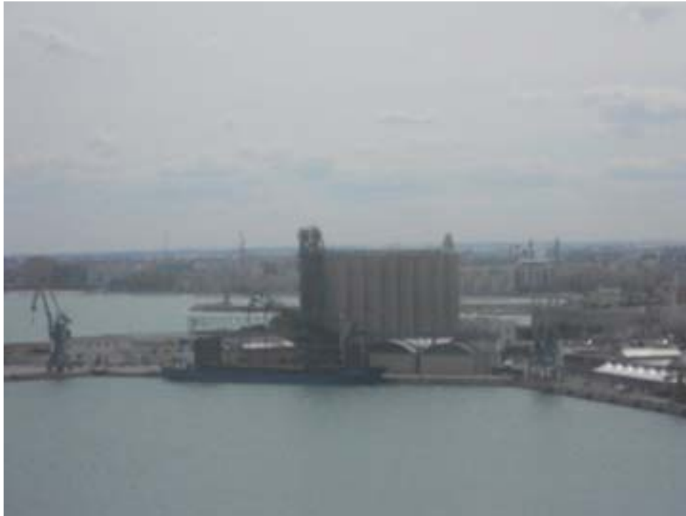
Grain Berth (Berth No. 15) and Silos in Darsena di Levante
