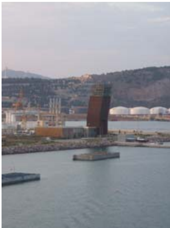
Barcelona—Harbor Control Tower
