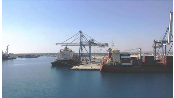
Limassol Container Terminal
