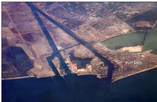
Port Sa'id (aerial view)
